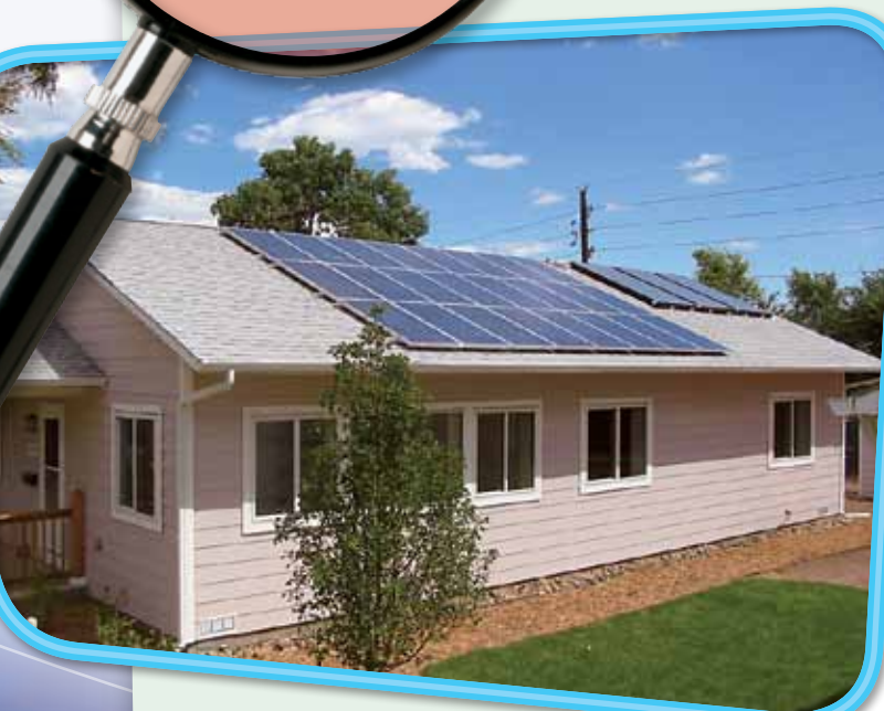
This zero-energy home in the United States uses passive solar design to reduce energy requirements for heating to a small fraction of the requirements of an average home.
